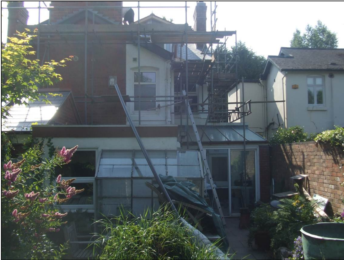
Figure 1 – 11 Harrison's Road rear elevation and boundary with No.13
