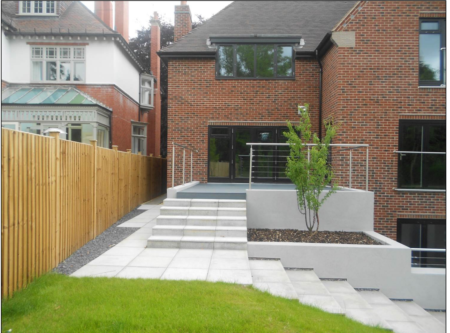
Figure 1 – View of raised decking area in relation to boundary with 17 Four Oaks Road
