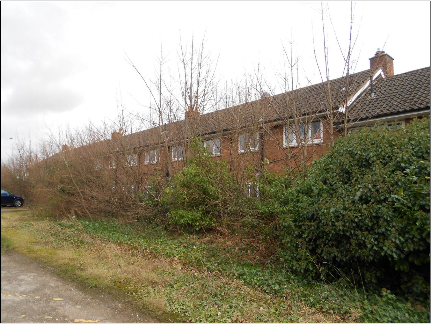
Figure 3 – Rear of properties in Mere Drive
