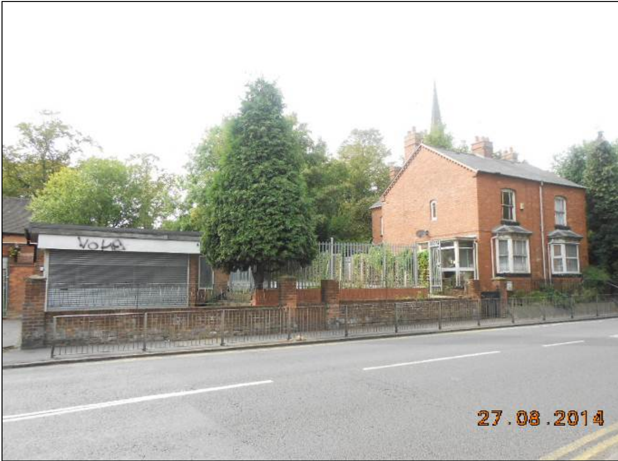
Existing dwellings to be demolished fronting Pershore Road South
