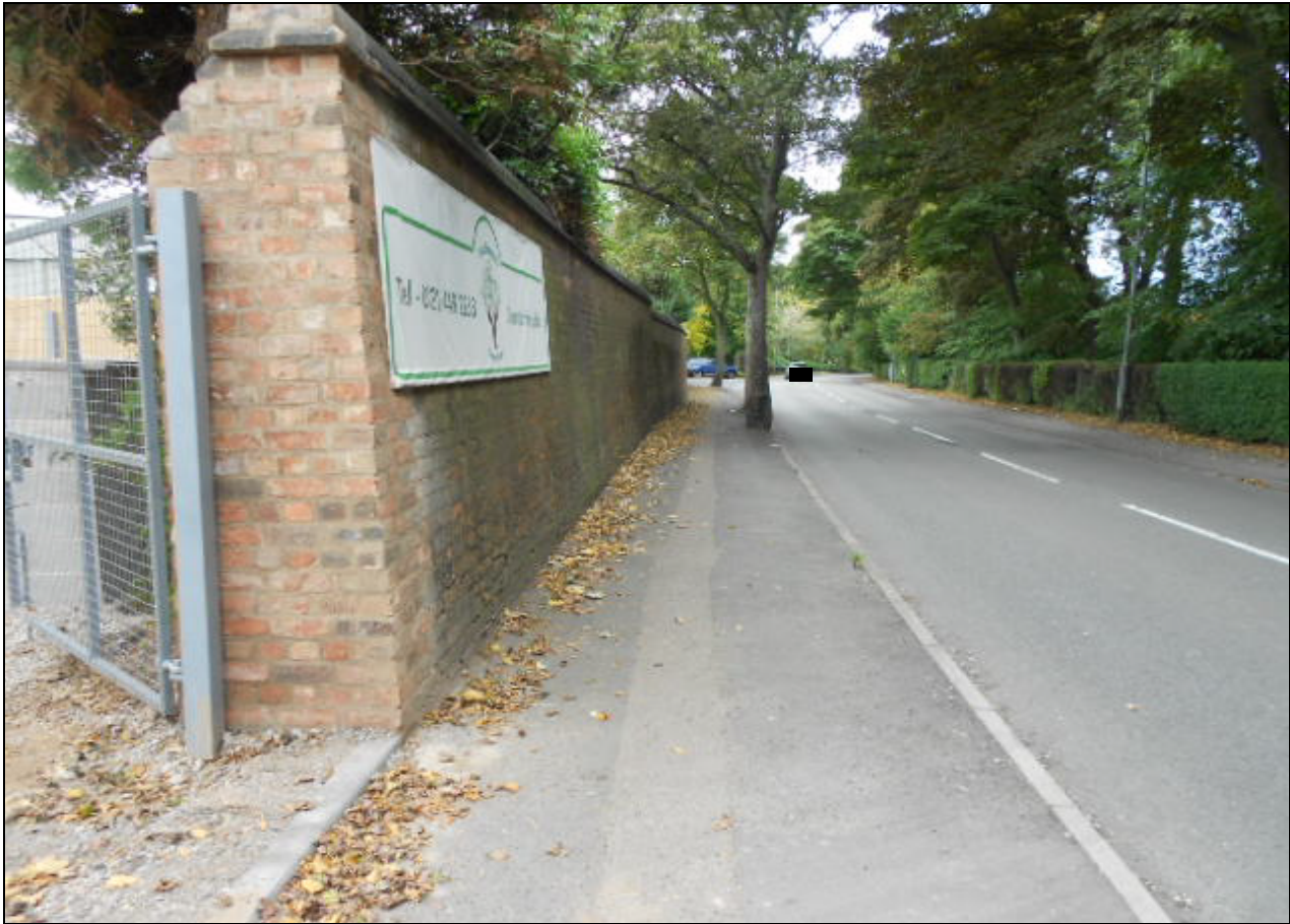
Figure 1 – Existing wall along Queensbridge Road
