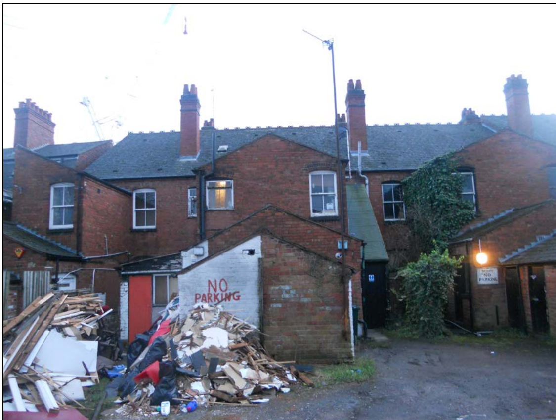
Figure 2 - Rear of application site
