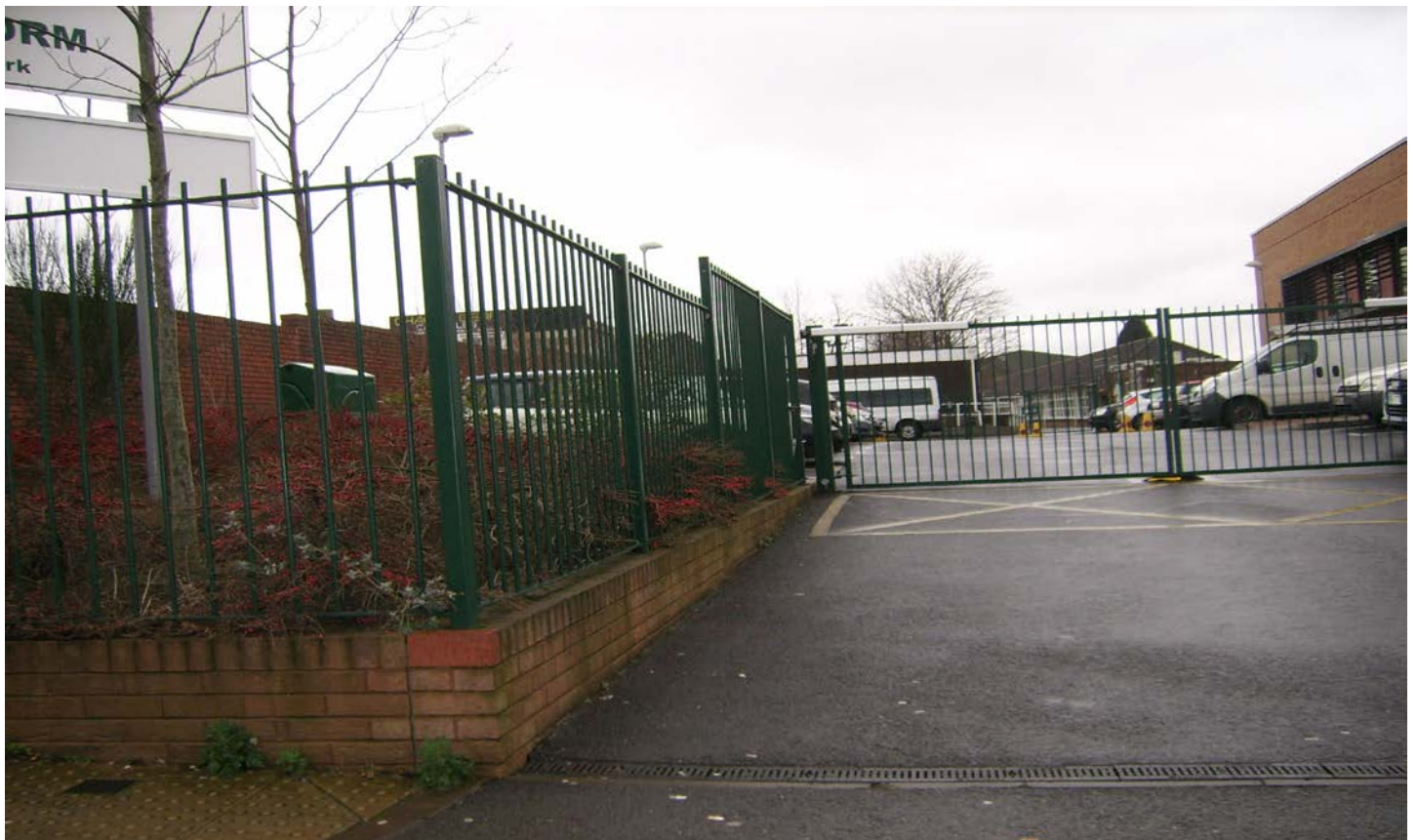
Figure 2: Street view of existing demountable building to be replaced
