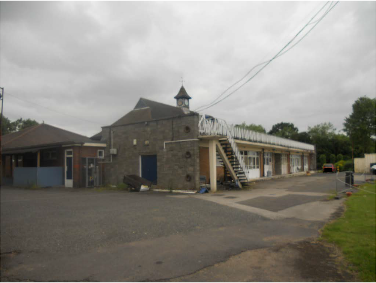
Fig1. View of existing pavilion
