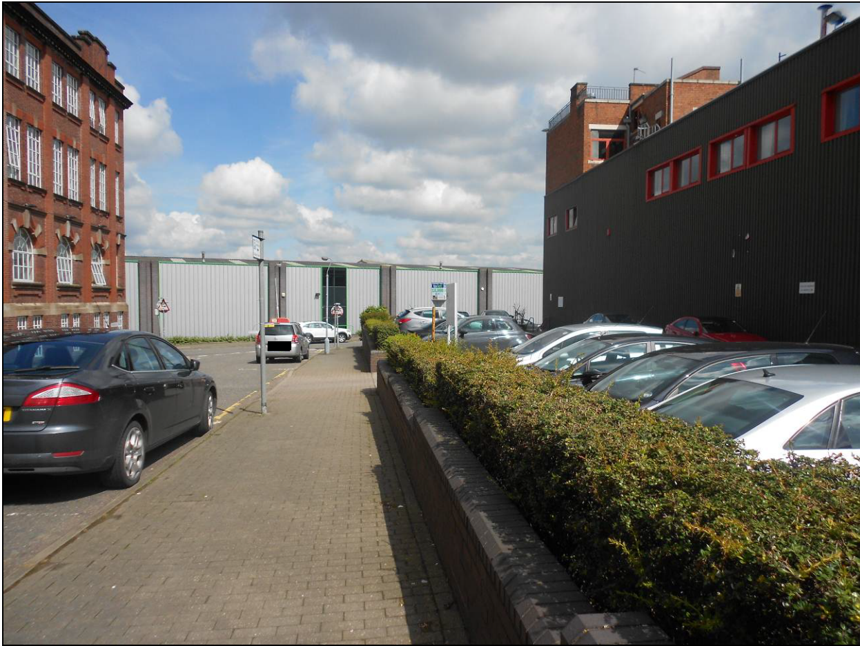
Figure 3: Side elevation opposite the Listed Pen Works
