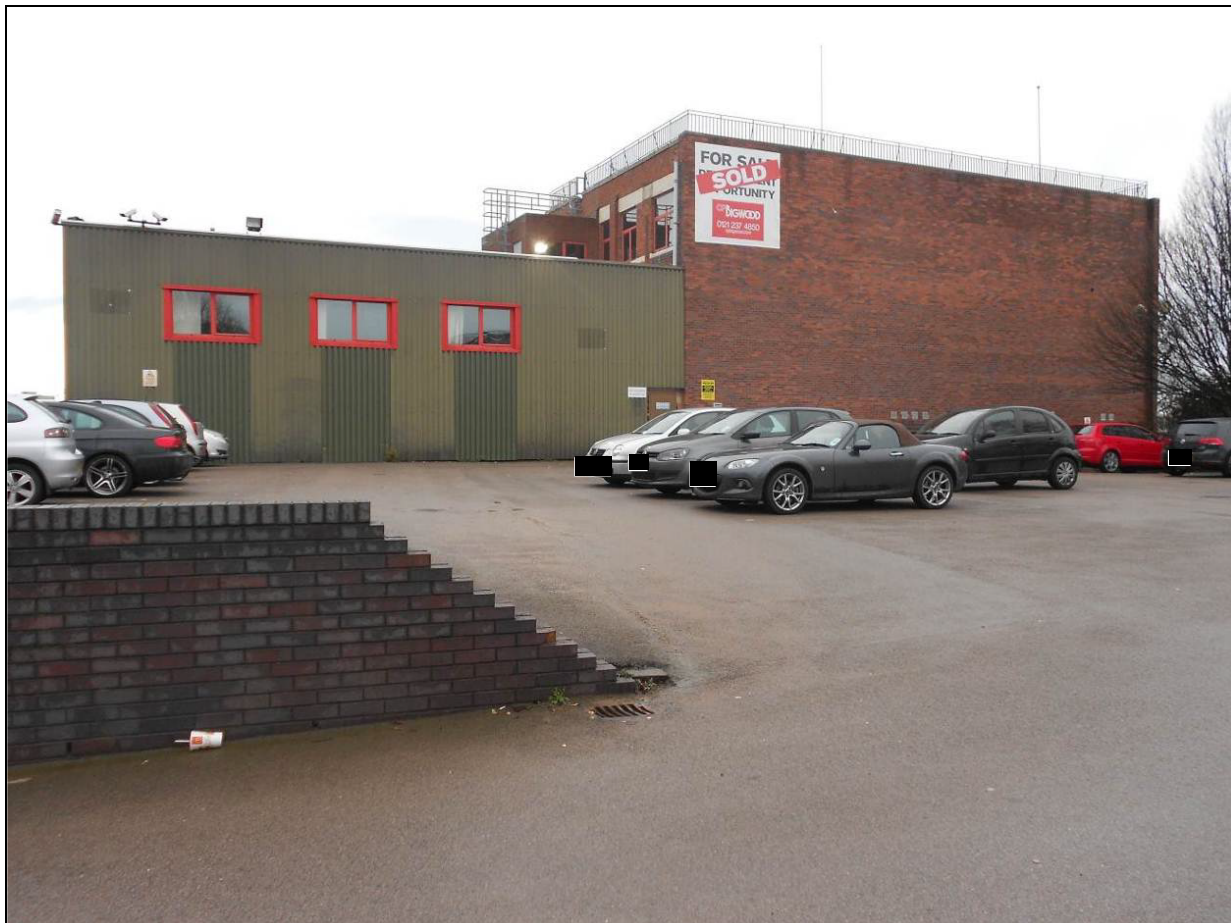
Figure 2: View to the rear of the existing building
