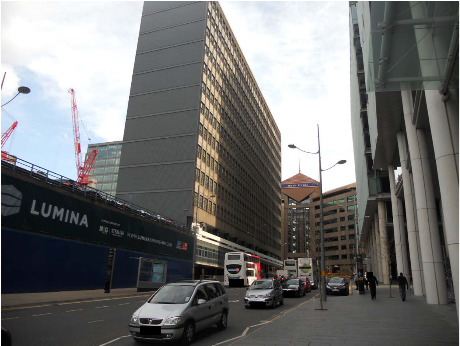
View along Snow Hill Queensway
