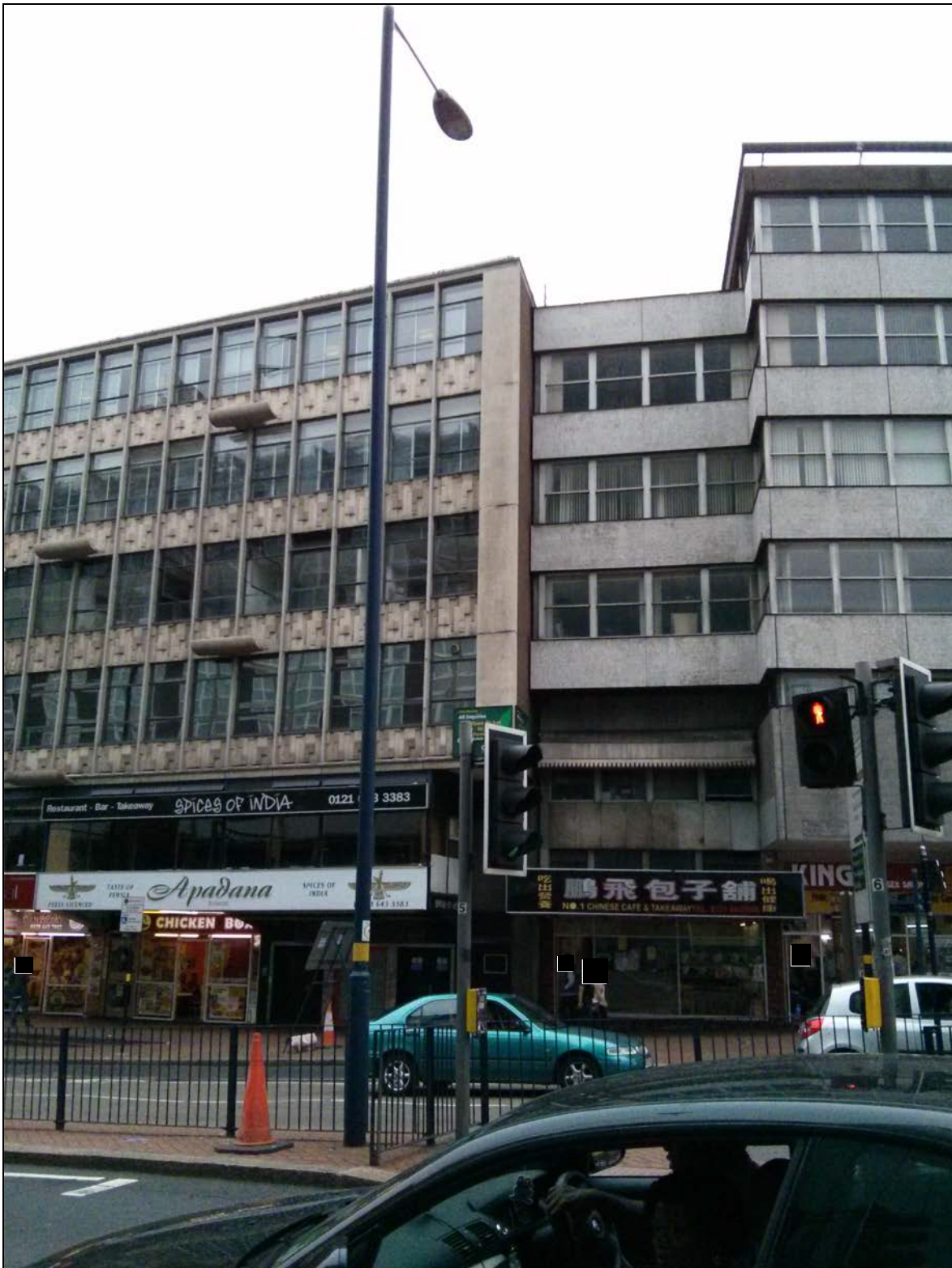
Figure 2 Junction with Locally Listed Building
